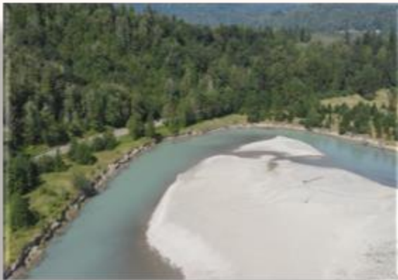
Concrete-Sauk valley Road M.P. 3.7
